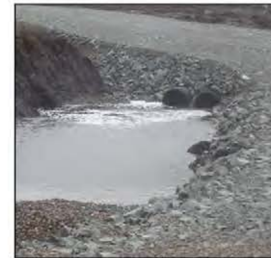
TYPICAL UNDER TRACK DRAINAGE
