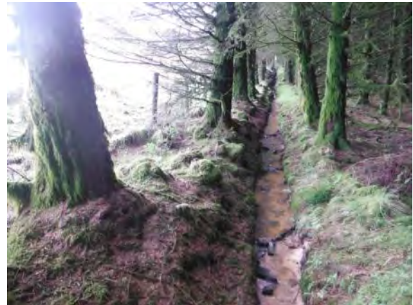
Drain intercepting upgradient groundwater at upgradient edge of forestry
