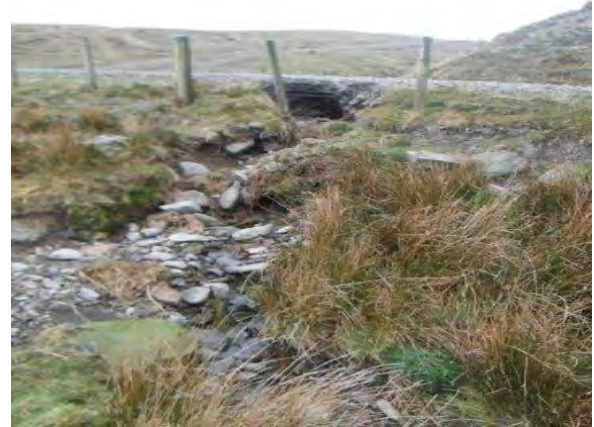
Photo 13. Water crossing 13: East access track over existing drain (SH 97030 07130)
