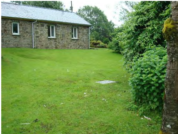
Photo 9. Private water supply for Ffridd Fawr (PWS 9)
