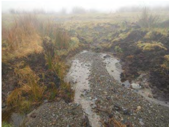
Photo 42. Existing drains at water crossing 17 on Afon Gam tributary (SH 94380 05580).
