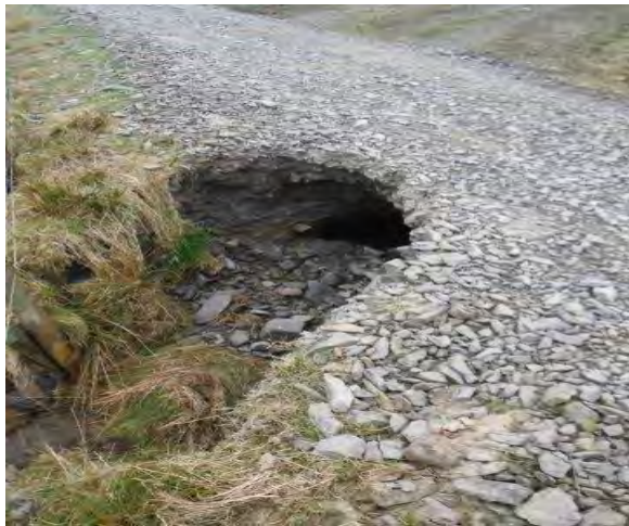
Photo 12. Water crossing 1: East access track over existing drain (SH 97030 07130)
