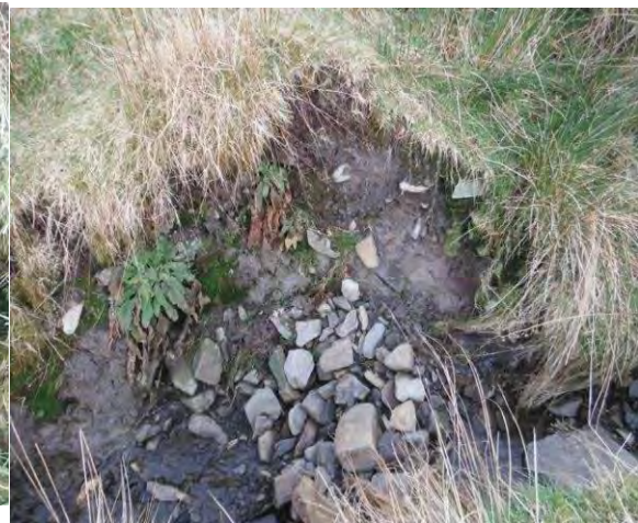
Photo 39. Bed of proposed water crossing 15 on Nant y Graig Lwyd tributary
