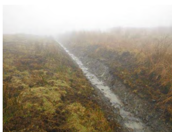
Photo 41. Existing drains on Afon Gam tributary at water crossing 16
