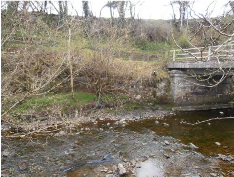
Photograph 3 - River Bank to west at Gosen Bridge, Afon Gam river crossing
