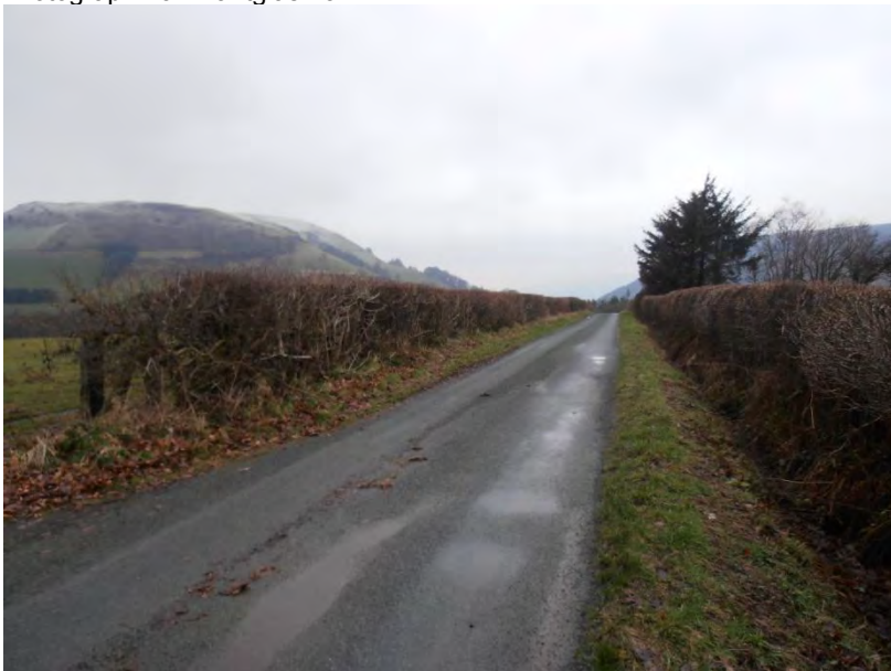
Photograph 20 - Road narrowing with hedgerows at Chainage 17,075
