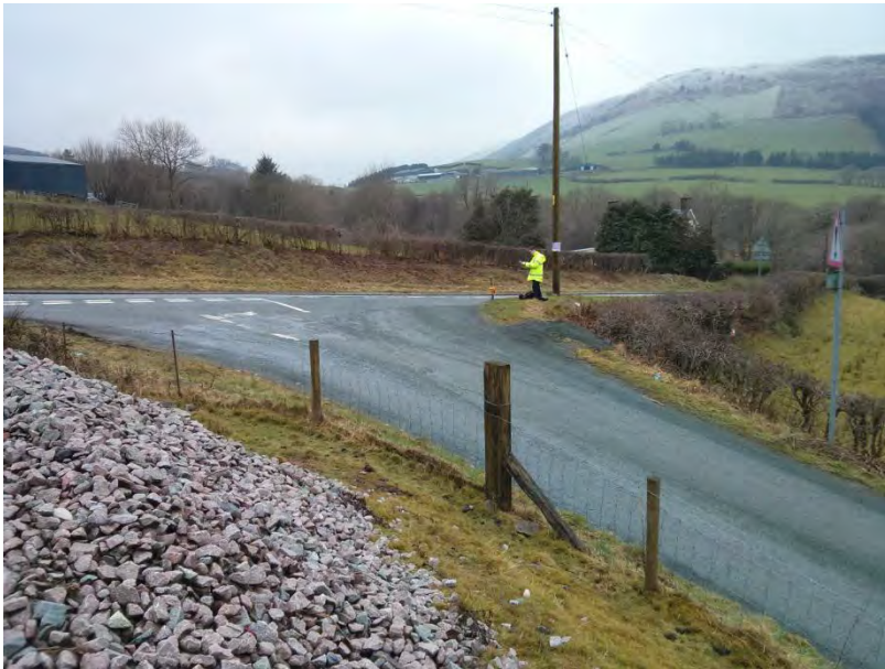
Photograph 21 - Talerddig Junction from Highway Depot to the east of the junction.
