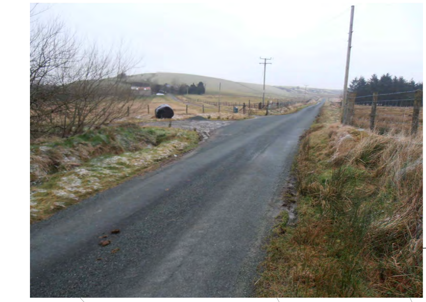
3.13 - EXISTING PASSING AREA AT ACCESS CH 15350 EXISTING PASSING PLACE AREA BETWEEN THE TWO JUNCTIONS IS OF SUFFICIENT SIZE TO ACCOMMODATE HOVS.
