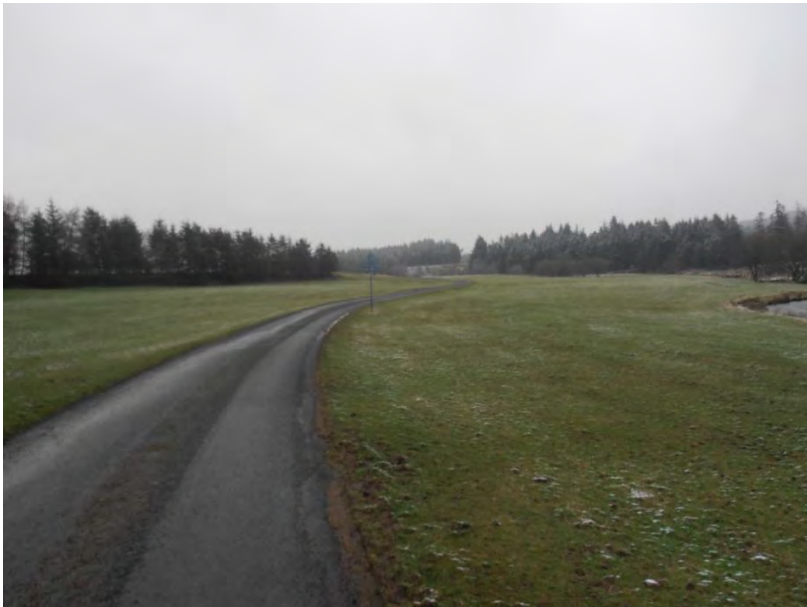
Photograph 15 - Existing Road between Access 2 and 4, at Chainage 11,400.
