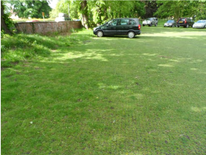
Photograph 24 - Grass Reinforcement at the University of York, approximately 18 months old
