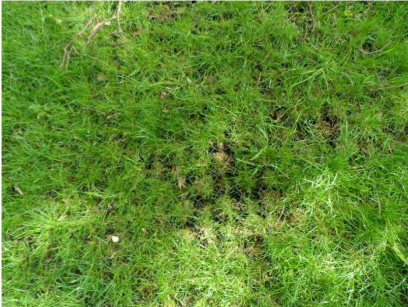
Photograph 23 - Grass Reinforcement at the University of York, approximately 18 months old.
