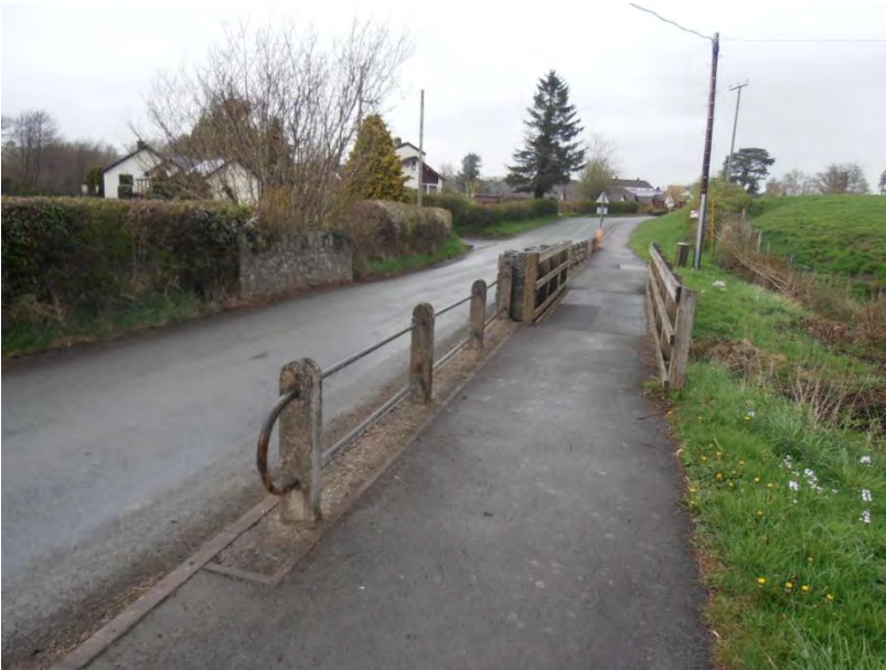
Photograph 2 - Glen Menial Bridge
