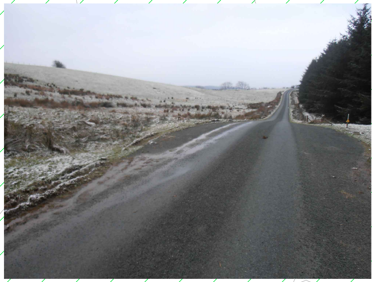
3.4 - NEW PASSING PLACE AT ACCESS CH 13840 THE BELL MOUTH OF THE EXISTING ACCESS JUNCTION IS TO BE WIDENED ON THE SOUTH-EASTERN SIDE USING GRASS REINFORCEMENT TO CREATE A PASSING PLACE FOR HGVs. ALL WORKS ARE TO BE CONSTRUCTED OFF-LINE FROM ADJACENT VERGE AREA WITH NO IMPACT ON EXISTING VEGETATION, DRAINAGE AND FENCE LINES.
