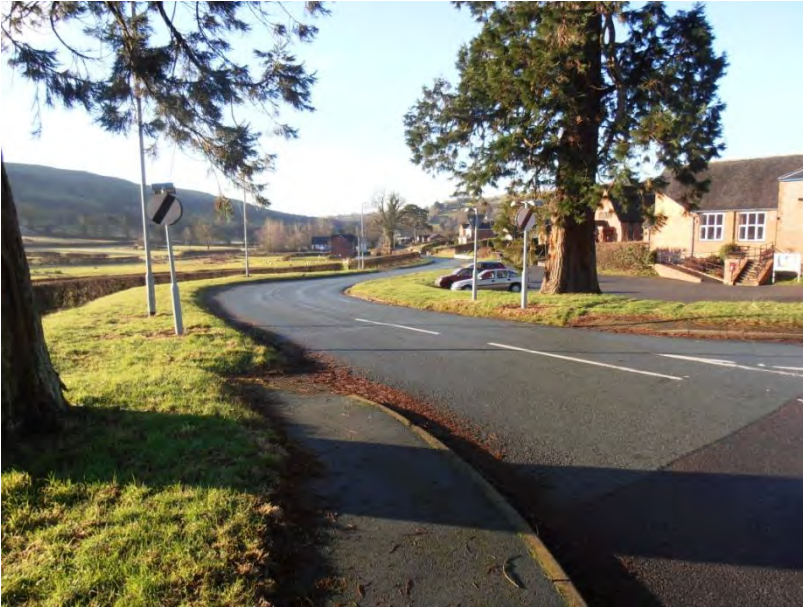
Photograph 1 - A458 / C2031 Junction at Llanerfyl
