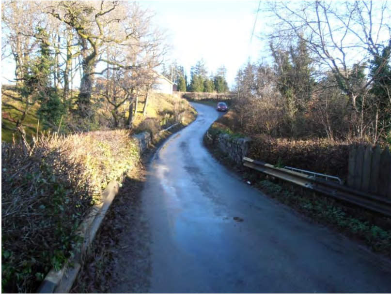
Photograph 4 - Gosen Bridge - Looking west to east. Bridge is in the foreground, Chapel is to the right of the picture. Afon Gam is to the left of the hedgerow in the left of the picture.
