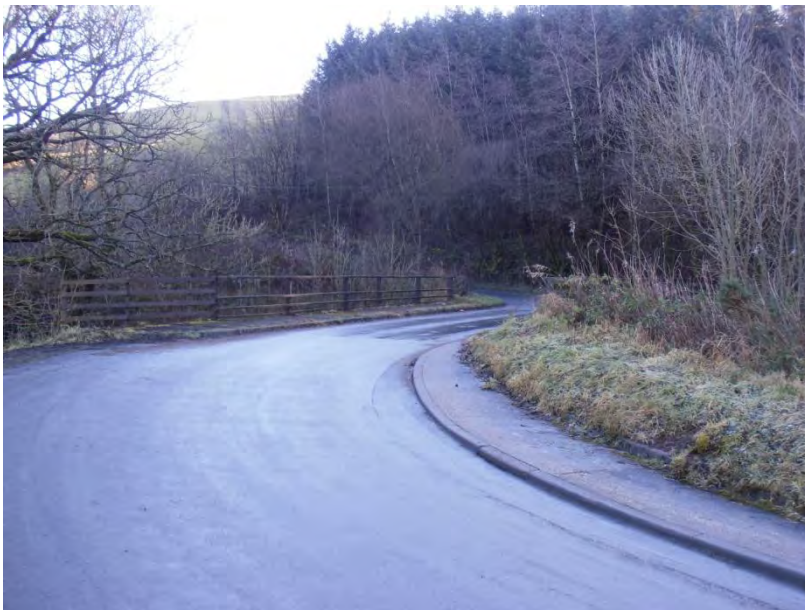
Photograph 8 - Dolwen Isaf Bridge
