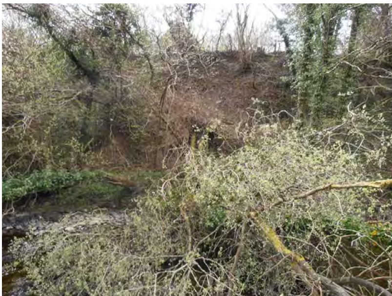
Photograph 2 - Tree Fallen on embankment to west of Gosen Bridge, opposite Gosen Chapel
