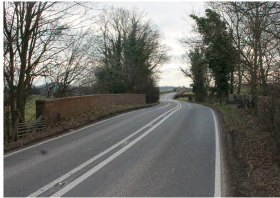
Figure 3-2 - Bridge over Dismantled Railway (South of Pont Rhyd-Meredydd)
