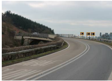
Figure 2-2 - Railway Bridge at Trewern
