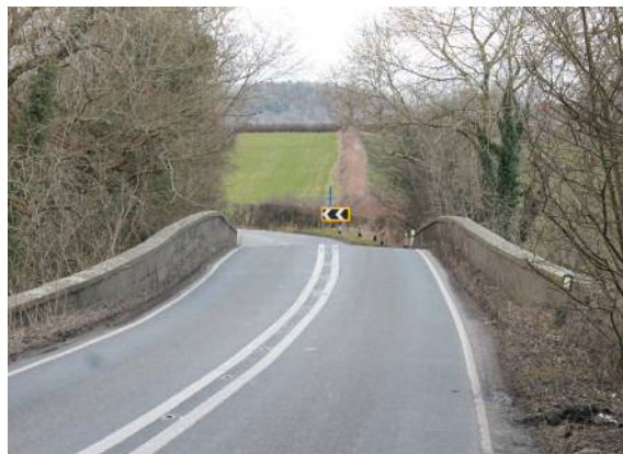
Figure 3-1 - Bridge over Afon Tanat
